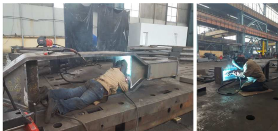
Fig. 1. Welding positions from factory [author’s photos].
