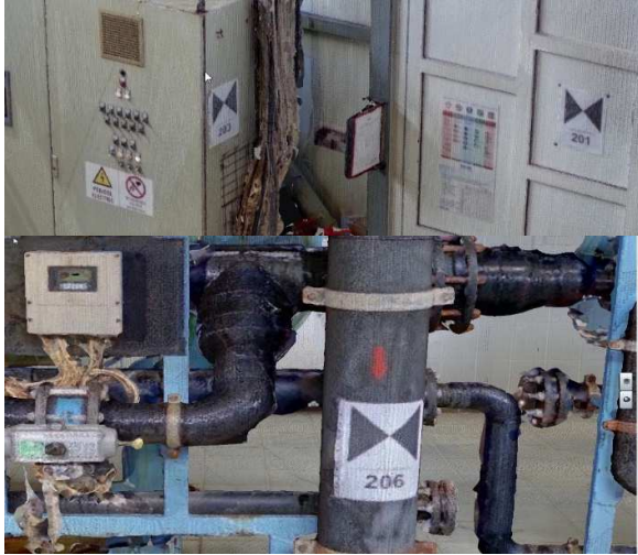
Fig. 3 Target used in TLS
