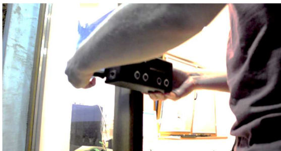
Fig. 10. Installing the device on site
