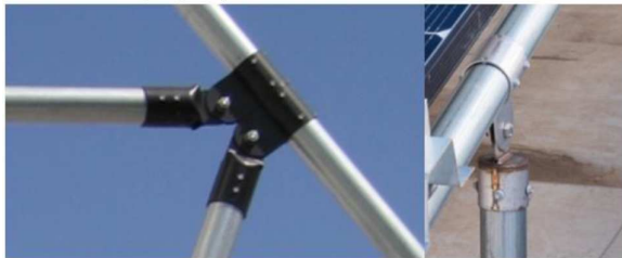
Fig. 2. Assembly using connector fittings adapted to the shape of the tubes [1] [2]
