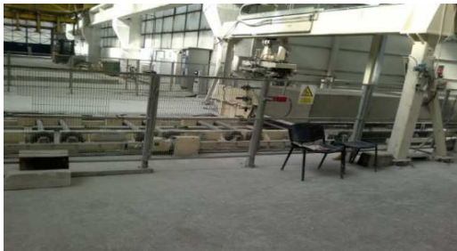
Fig. 3. Conveyor for transporting cut items.
