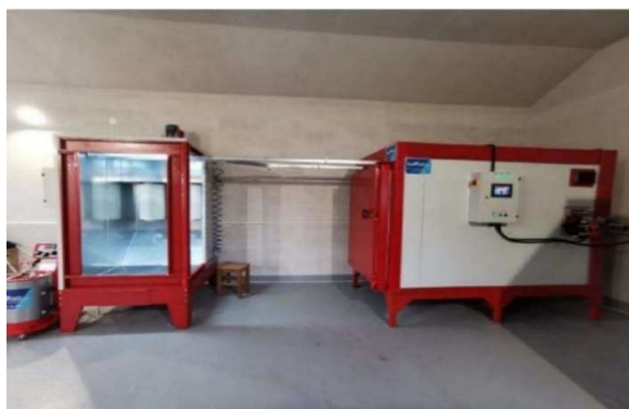
Fig. 3. Painting working area
