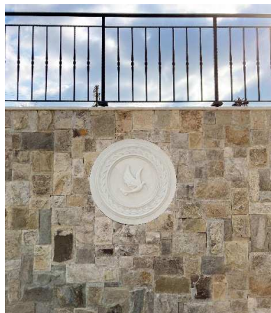
Fig. 8. Casting of a dove made out of concrete
