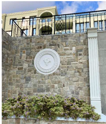
Fig. 7. Casting of a grape relief, built in next to a pilaster in same the style
