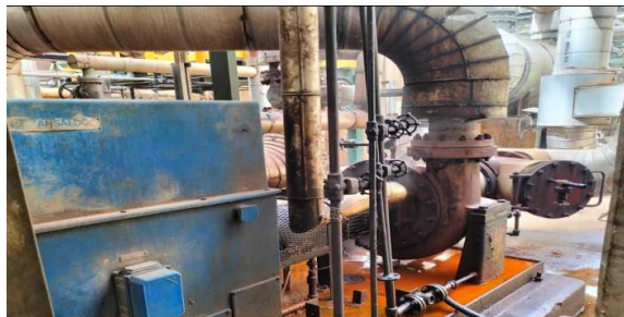
Fig.1. Photo of the installation of our machine.
