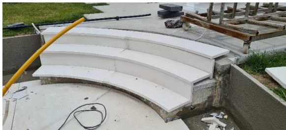
Fig.8. Steps cast in molds made using a vacuum-forming machine
