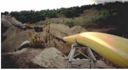
Fig. 2.2 Changing of pipeline section (photo Transgaz S.A.)
