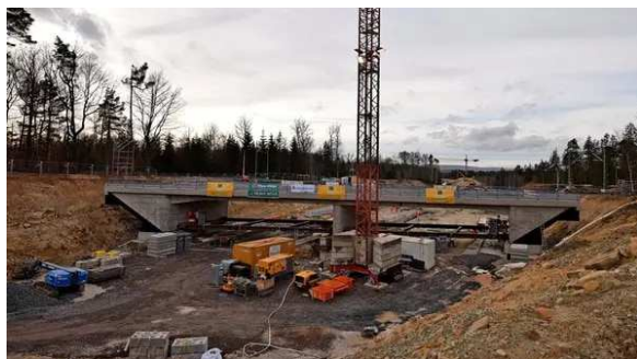
Figure 1. Concrete bridge construction site for the federal highway A49 [23]
