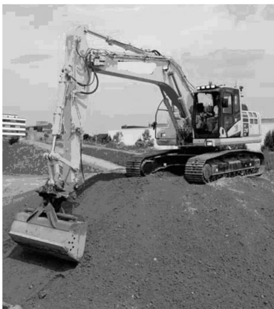
Fig.1. A hydraulic excavator with backhoe attachment used for leveling
