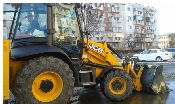
Fig. 1. Excavator with the pneumatic hammer
